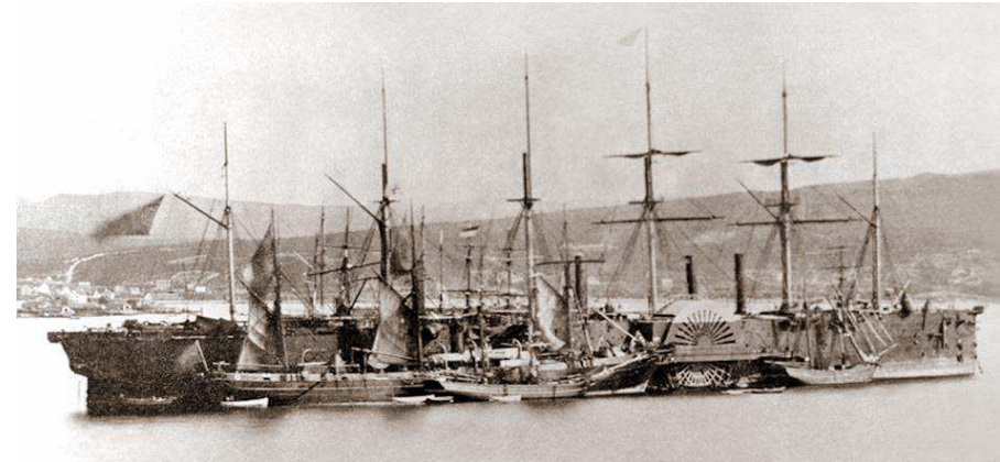
SS Great Eastern (1859) - Based on her trial voyage, Froude proposed the usage of bilge keels (Perez, 2005)
