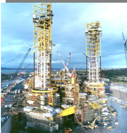
Fabrication in dry dock
