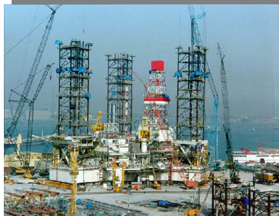
Fabrication on quay
