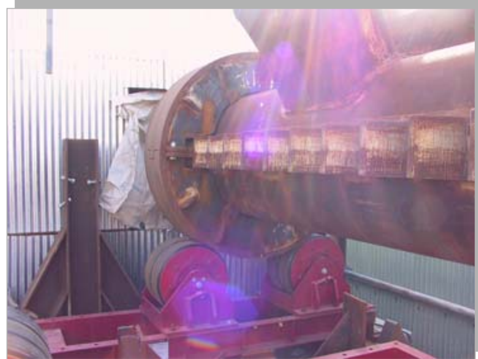
RACK TO RACK WELDING
