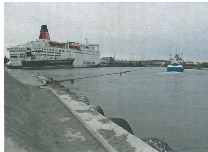
Bollard Pull Measurement in Frederikshavn
